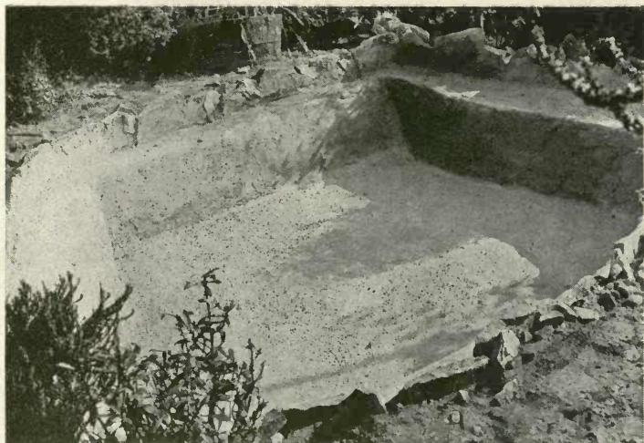
A LITTLE GARDEN POOL MADE WATERTIGHT WITH CEMENT
